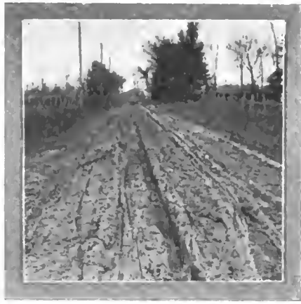
International road near St. John's, P. Q., before scraping
